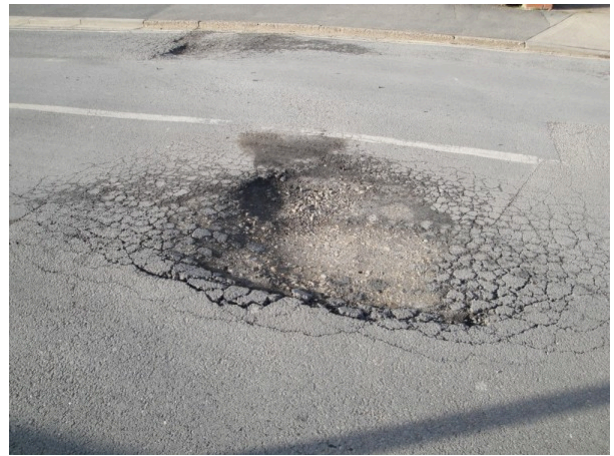
Figure 5. Thermal stress contributes to the formation of potholes. (credit: Editor5807, Wikimedia Commons)
