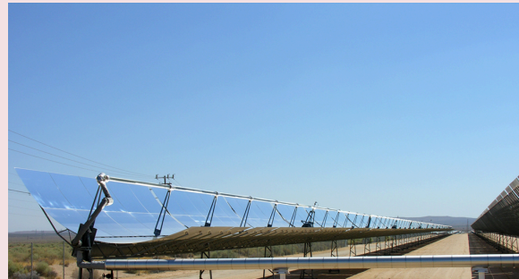
Figure 5. Parabolic trough collectors are used to generate electricity in southern California. (credit: kjkolb, Wikimedia Commons)
