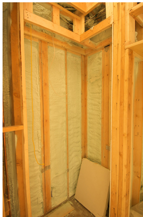
Figure 1. Insulation is used to limit the conduction of heat from the inside to the outside (in winters) and from the outside to the inside (in summers). (credit: Giles Douglas)
