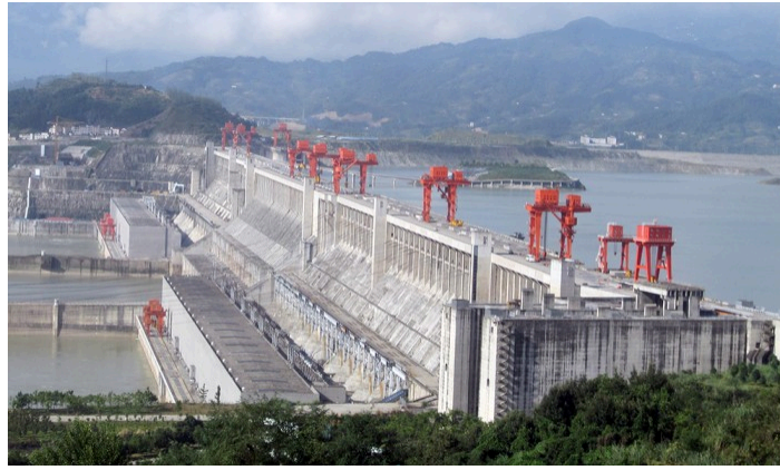
Figure 2. Three Gorges Dam in central China. When completed in 2008, this became the world's largest hydroelectric plant, generating power equivalent to that generated by 22 average-sized nuclear power plants. The concrete dam is 181 m high and 2.3 km across. The reservoir made by this dam is 660 km long. Over 1 million people were displaced by the creation of the reservoir. (credit: Le Grand Portage)
