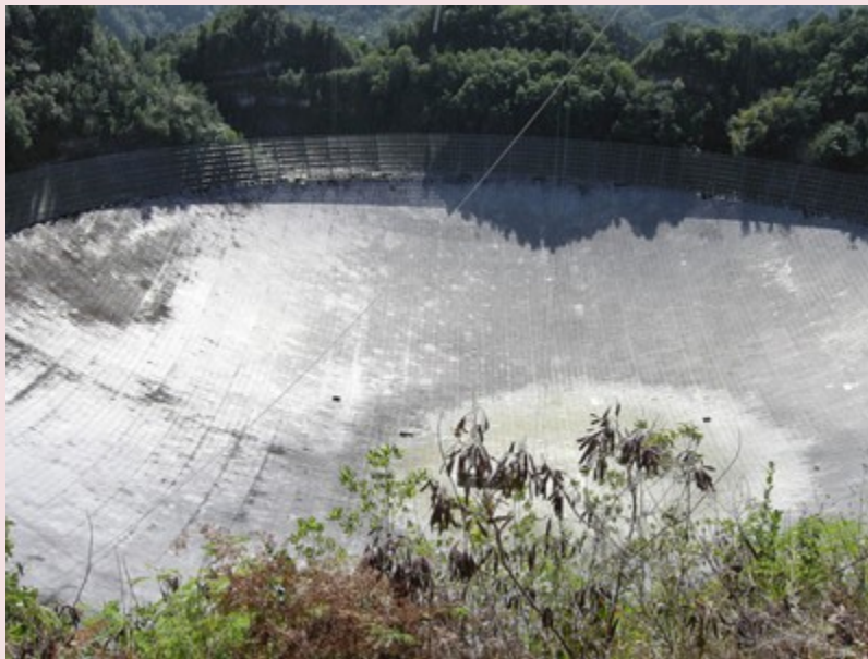
Figure 4. A 305-m-diameter natural bowl at Arecibo in Puerto Rico is lined with reflective material, making it into a radio telescope. It is the largest curved focusing dish in the world. Although D for Arecibo is much larger than for the Hubble Telescope, it detects much longer wavelength radiation and its diffraction limit is significantly poorer than Hubble's. Arecibo is still very useful, because important information is carried by radio waves that is not carried by visible light. (credit: Tatyana Temirbulatova, Flickr)
