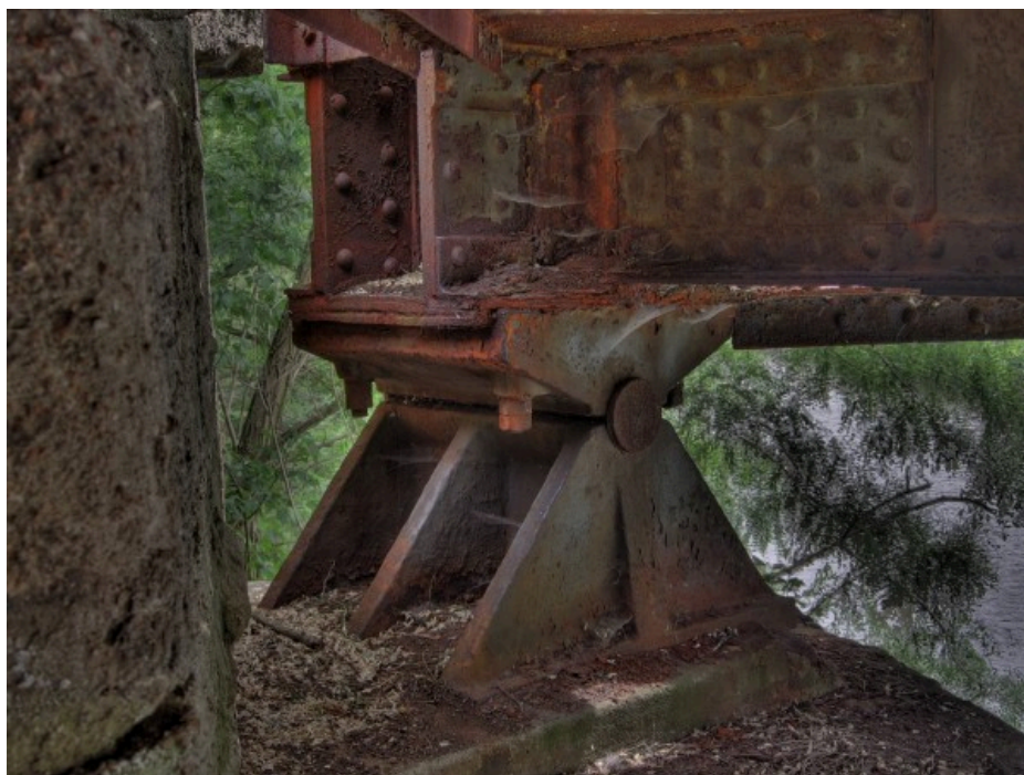
Figure 16.1 These support beams on a bridge are obviously rusted. If the rusting becomes too bad, it will compromise the integrity of the bridge, requiring replacement. Source: “rusty bridge bearing” by Fabian is licensed under the Creative Commons Attribution-NonCommercial-ShareAlike 2.0 Generic
