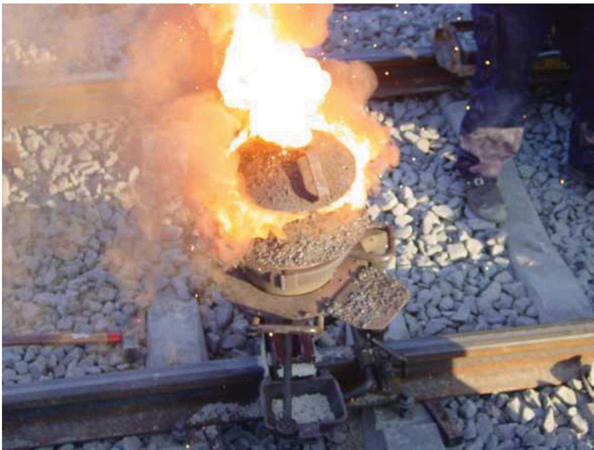
Figure 8.2 “Thermite Reaction.” A small clay pot contains a thermite mixture. It is reacting at high temperature in the photo and will eventually produce molten metal to join the railroad tracks below it. Source: Photo courtesy of Skatebiker, http://commons.wikimedia.org/wiki/File:Velp-thermitewelding-1.jpg .
